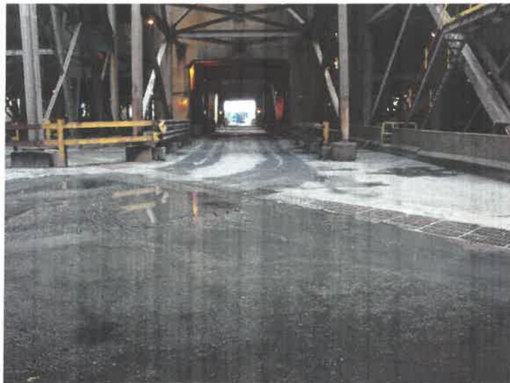
Mt. Storm Station Reinforced Concrete Pavement
