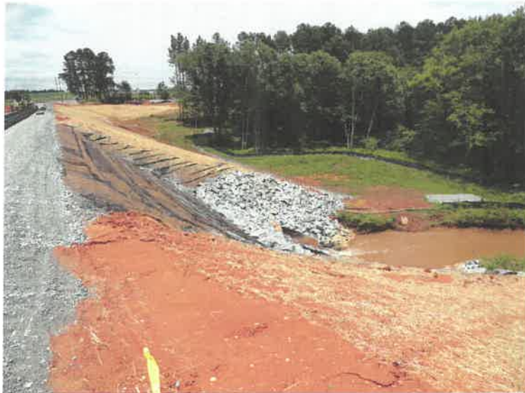
Reinforced Soil Slope around Twin Culverts.
