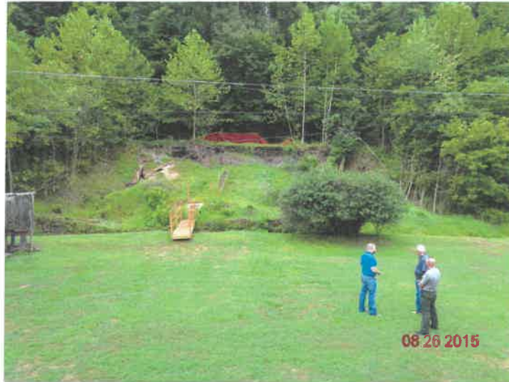
Overview of NBRT Landslide
