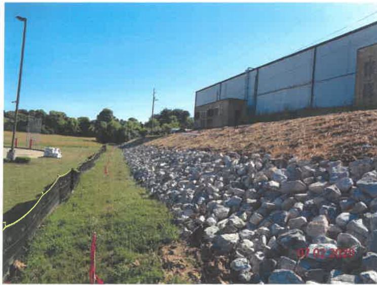
Buttress and Rock Toe Construction to Stabilize the Slope
