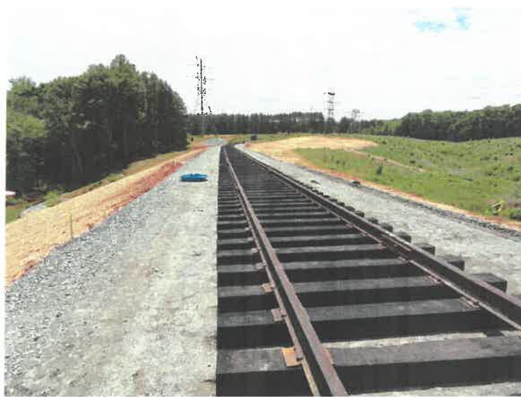
Improved Subgrade and Rail System.
