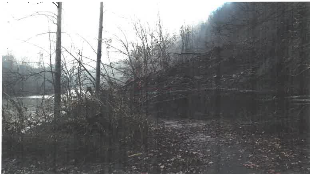
GBRT Blocked by Slide
