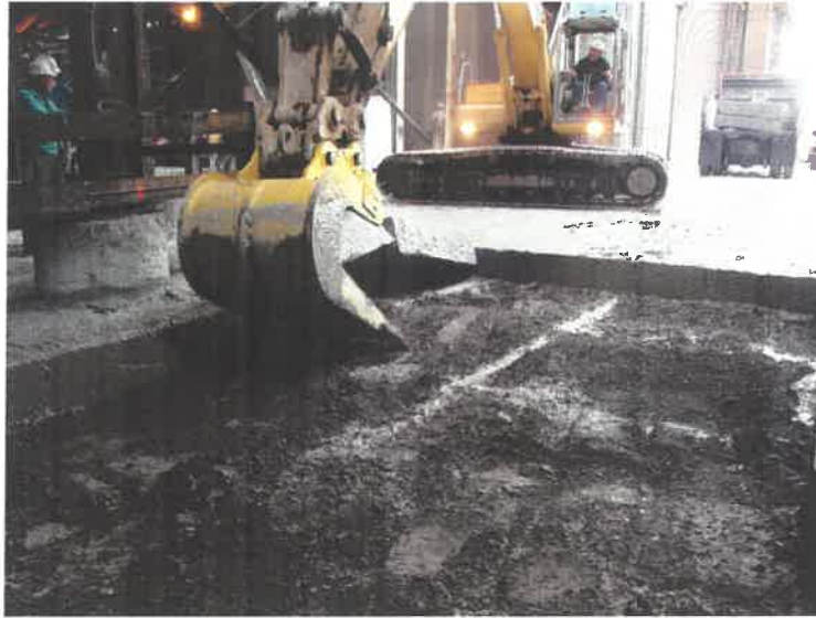
Removing Old Pavement from Mt. Storm Station
