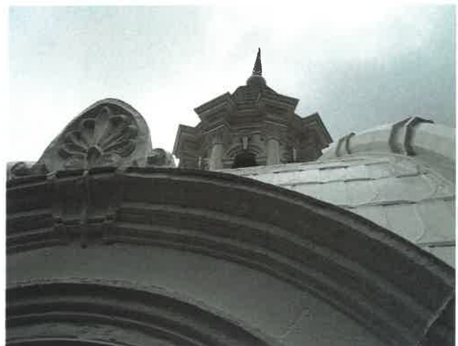
Dome Restoration Detail
