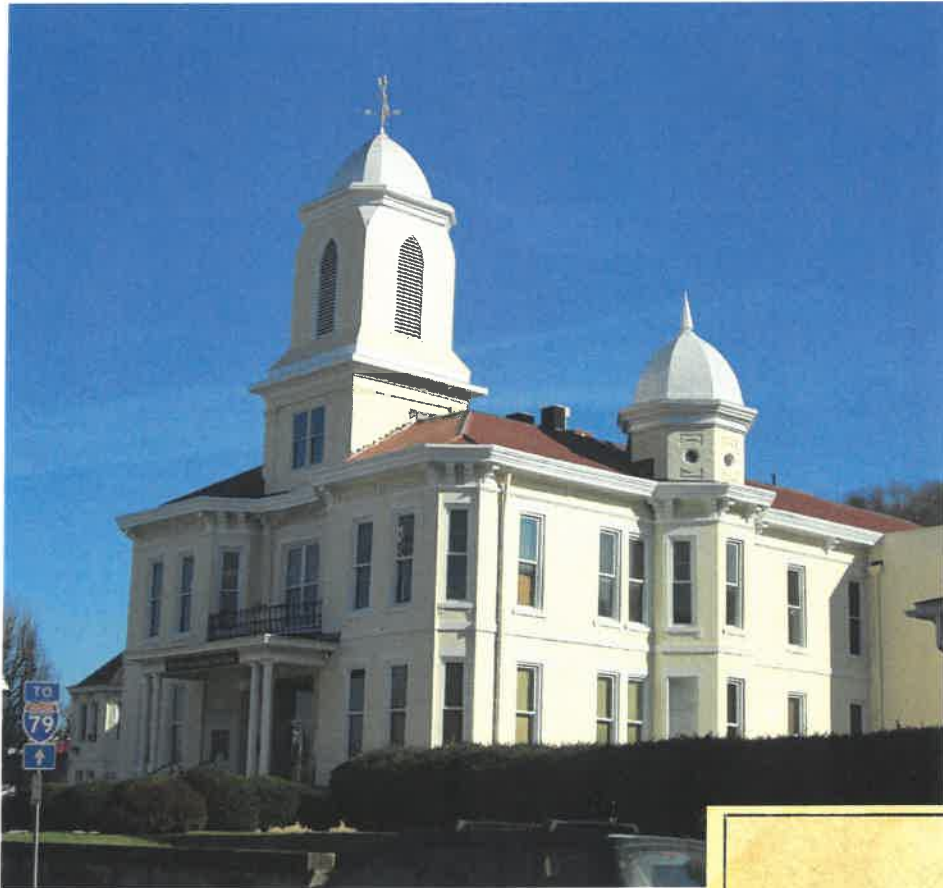
Lewis County Commission Courthouse Conditions Report/Roof Restoration 18 Garton Plaza Weston, West Virginia
