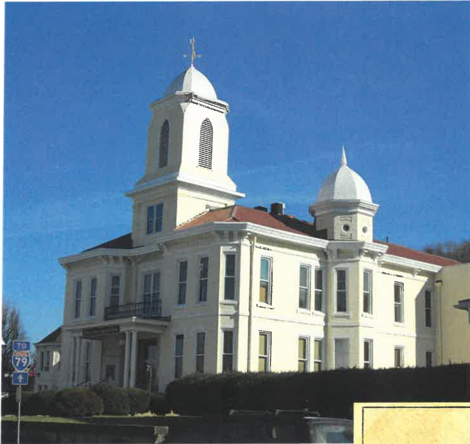
Lewis County Commission Courthouse Conditions Report/Roof Restoration 18 Garton Plaza Weston, West Virginia
