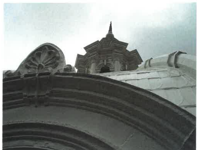
Dome Restoration Detail
