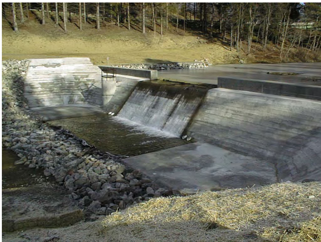
THOMAS DAM MODIFICATION, THOMAS, WV
