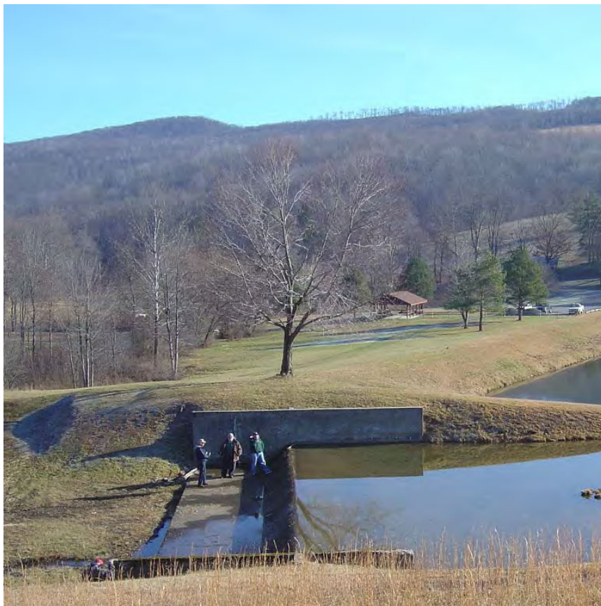
BELINGTON DAM MODIFICATION, BELINGTON, WV
