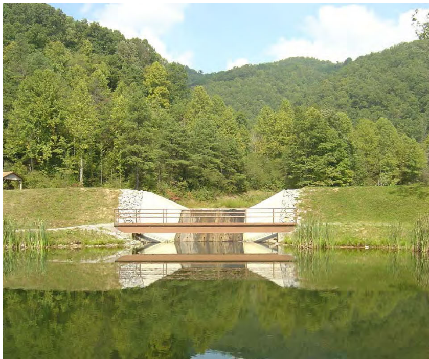
OLD ANAWALT DAM FLOOD DAMAGE REPAIR, MCDOWELL CO., WV
