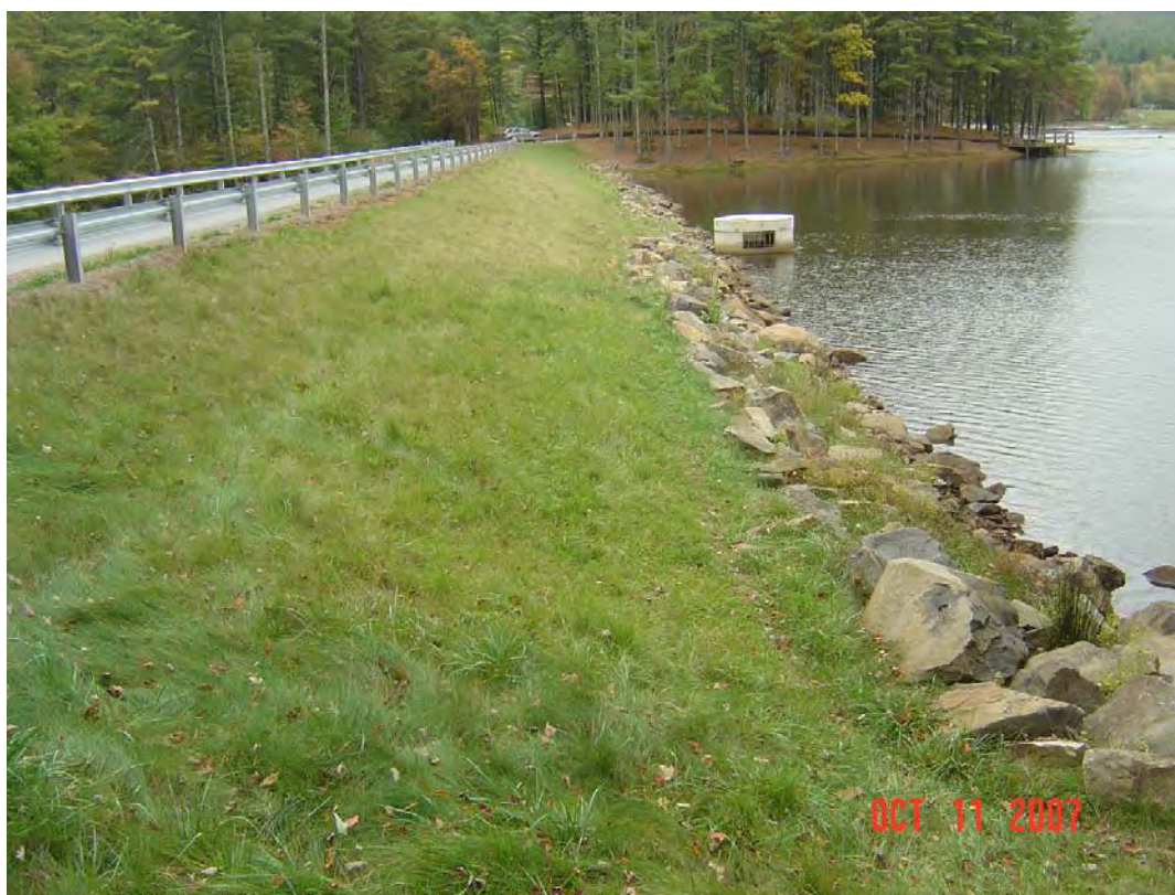
MONCOVE DAM MODIFICATION, MONROE CO., WV
