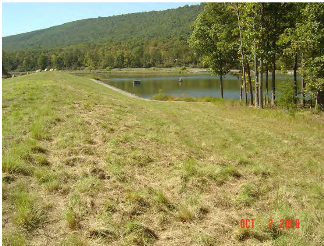
WARDEN LAKE DAM MODIFICATION, HARDY CO., WV
