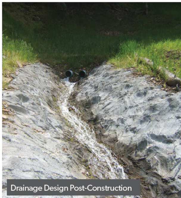
Drainage Discharging into a Stormwater System
