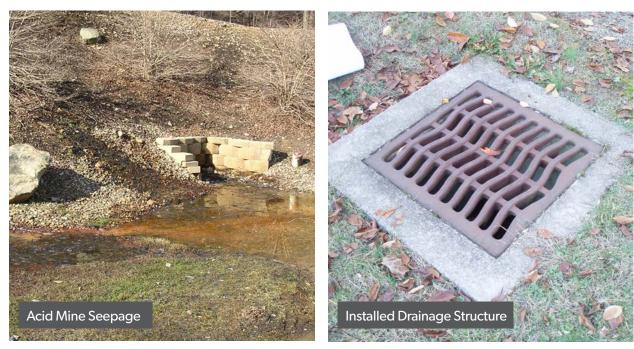
GAI provided engineering services to the West Virginia Department of Environmental Protection, Office of Abandoned Mine Lands and Reclamation for the Greystone Mine Drainage Project, located near Cheat Lake, Monongalia County, West Virginia. Acid Mine Drainage seepage from the highwall benches is causing hot spots in lawns and driveways and has caused flooding during heavy precipitation events.
