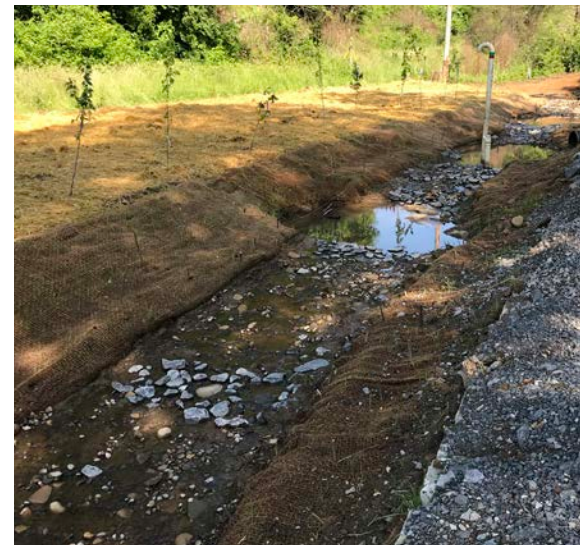
Impacted Stream Post Construction
