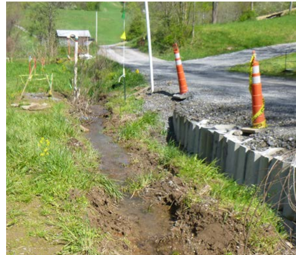
Impacted Stream Before Construction
