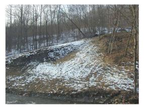
stability analyses were performed to determine the corrective actions required to stabilize the area. Surface and subsurface drainage structures, a toe key, and stream bank protection were designed to correct the instability problems and provide long term protection to the area.
