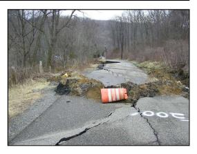
Site design will begin on the collection and diversion of ground water, slope stability and road replacement once the final site investigation has been completed.
