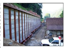
rock anchor tie-back system due to mine voids existing at the base of the hillside slope that were encountered during the subsurface exploration.
