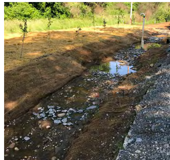
Impacted Stream Post Construction
