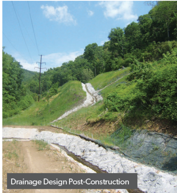
Drainage Discharging into a Stormwater System
