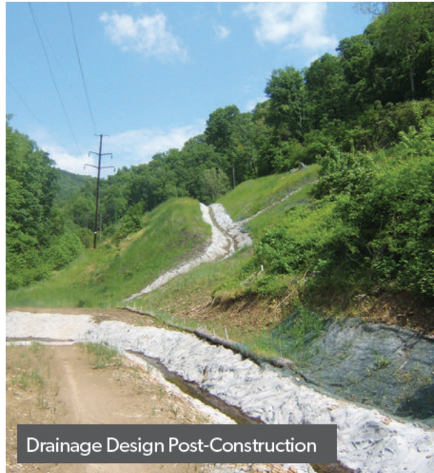
Drainage Discharging into a Stormwater System
