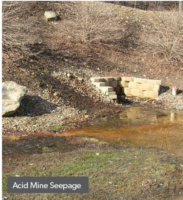
Installed Drainage Structure
