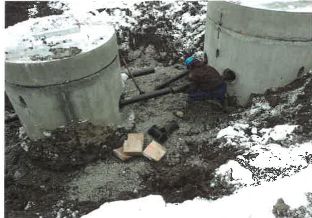
Lift Station Improvements
