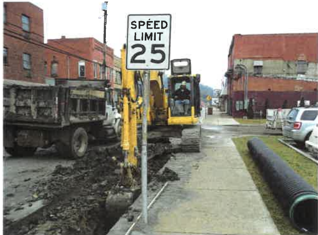
Storm Water Separation on US Route 250
