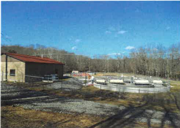
New 0.370 MGD WWTP
