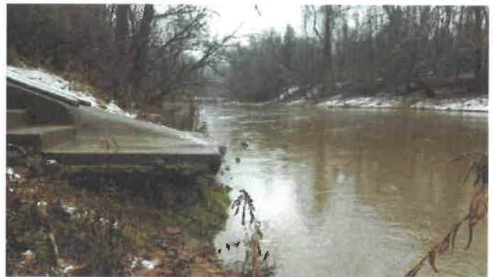
Snyder-Route 19 Public Fishing and Boating Access Site de-watered boat side. West Fork River is approximately three feet higher than normal in the photo.
