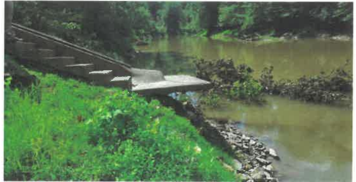
Route 36 Public Fishing and Boating Access Site de-watered concrete boat slide.
