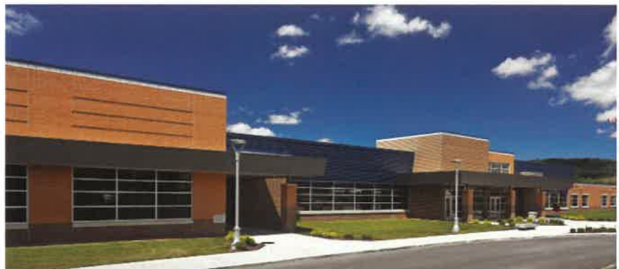
Above: Front facade of the Suncrest Elementary School located in Morgantown, WV. This project was designed incorporating sustainability concepts and focusing on the STREAM curriculum. (Science/Technology/Reading/Engineering/Art/Math)
