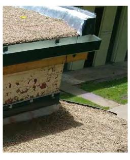
West Virginia Division of Natural Resources contracted Montum Architecture to specify and administer roofing replacement of the Pool Bathhouse at Berkeley Springs State Park. The existing roofing was a combination of EPDM and built-up roofing. Failing wood framing was replaced and ACM abatement was incorporated in the demolition.
