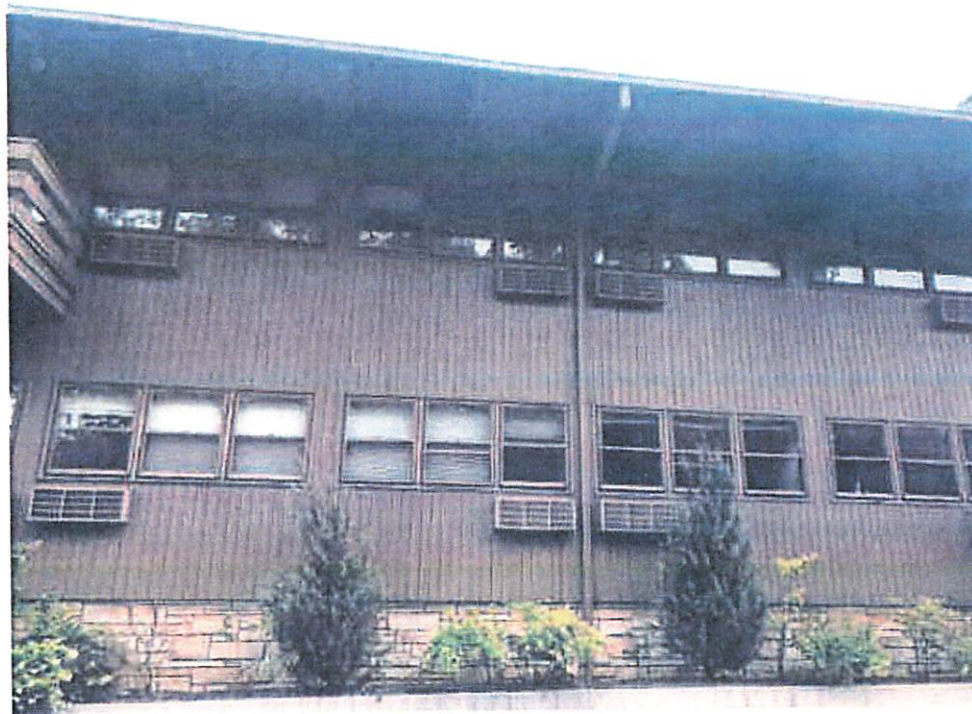
Photo 12: Downspout configuration back portion of rear of building (lake side).
