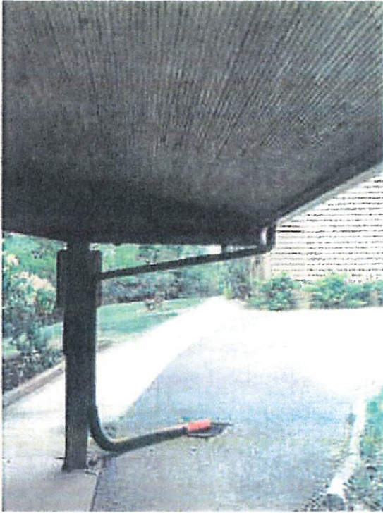
Photo 9: Downspout front corner of Activities Building.
