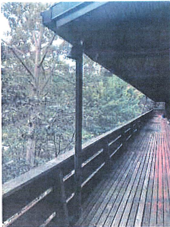
Photo 8: Downspout back of Activities Building Configuration 2.
