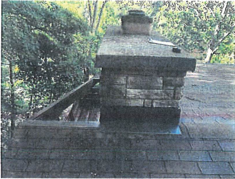
Photo 5: Chimney looking from side. Note portion of roof left open.
