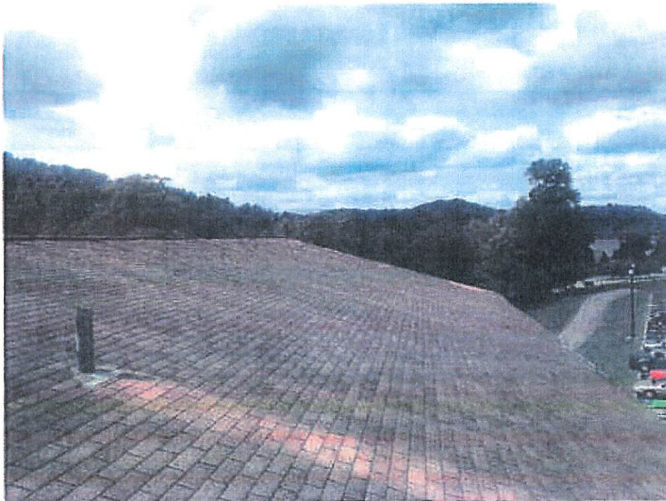
Photo 2: Main building roof looking from center near chimney towards front.
