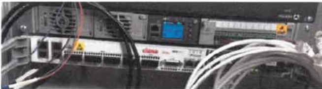
Installed equipment (switch and rectifier)
