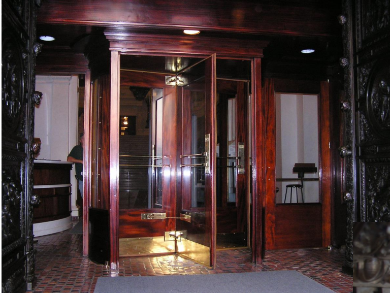
Restoration & Conservation of circa 1919 Mahogany Wood revolving Doors and Mechanisms at the PA State Capitol.
