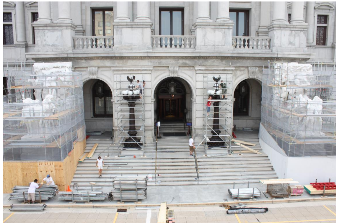
Erecting scaffold around the standards prior to treatment.
