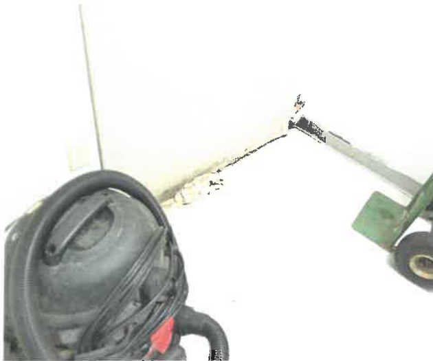
Water damage and mildew.
