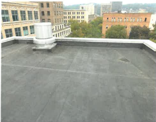
Roof and parapet caps.
