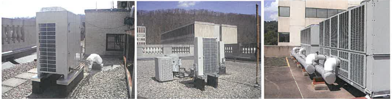
Old Kanawha Valley Bank Building (2003) - New cooling chiller. (2015) - New cooling tower.
