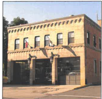
Central Fire Station
