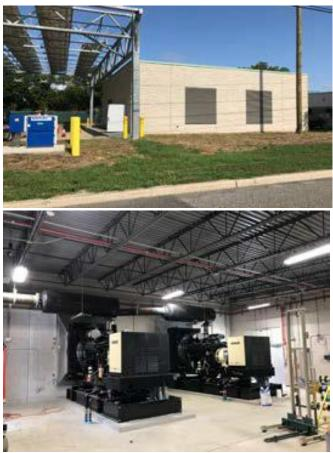
incorporates planned upgrades from the local utility authority which will be a transition from 4160 V to the 13.2 kV. Functional areas with the PPB include space allocation of the 2 generators with reserved interior floor space for future generator growth, and integration with alternate energy systems within the National Guard Training Center installation (Photovoltaic, wind, storage) using parallel switchgear and control interfaces.
