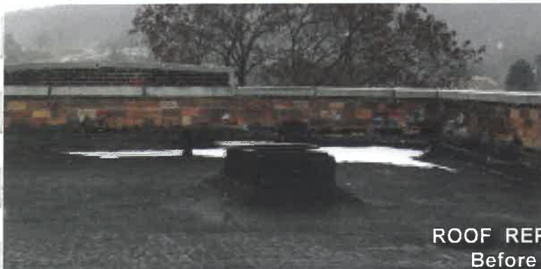
COPING AND PARAPET WALL UPGRADES Before & After
