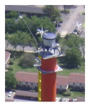
are either horizontally of elliptically polarized include a galvanized steel climbing pole for beacon access. All top mounted TRASAR antennas include four (4) lightning spurs at the top of the antenna.
