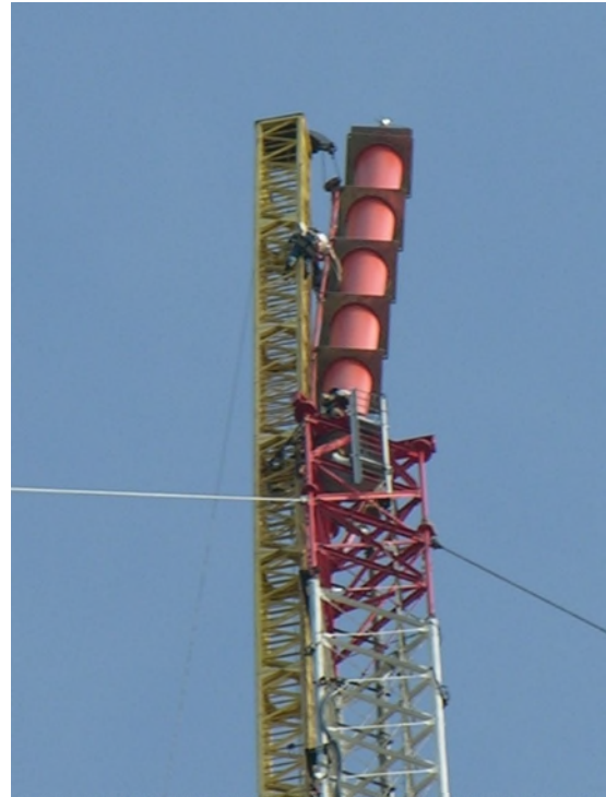
ERI TRASAR® High Band VHF Television Antenna. The antenna pictured is a circularly polarized. The antenna includes a fiberglass ladder for beacon access which has minimal impact on its omnidirectional azimuth pattern.
