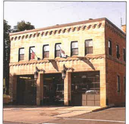
Central Fire Station
