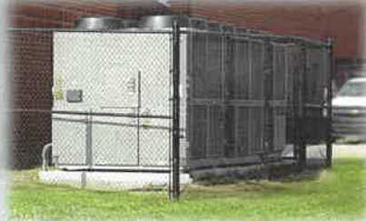
Chiller & Air Handling Unit Renovations
