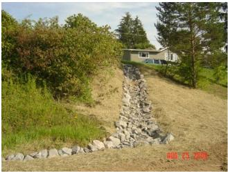
**Erosion Repair – Rip Rap Armored Ditch**
