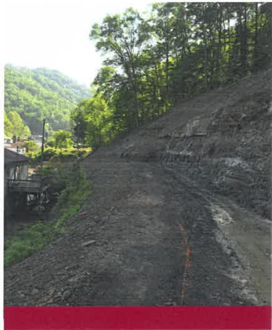
This project included 6,500 cubic yards of earthwork and stabilizing the slope behind the residence.
