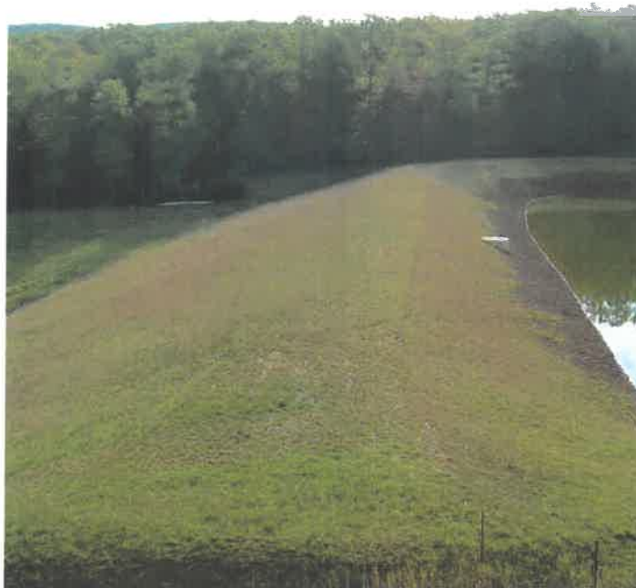
WILSON DAM MODIFICATION, HAMPSHIRE CO., WV
