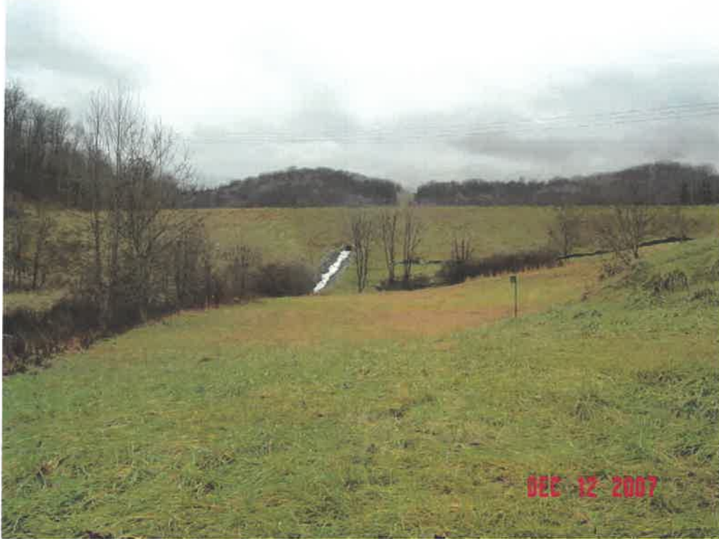
LEMLEY DAM MODIFICATION, MONONGALIA CO., WV
