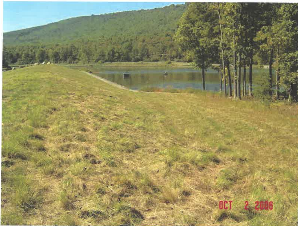
WARDEN LAKE DAM MODIFICATION, HARDY CO., WV
