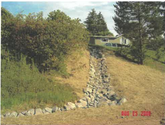
Erosion Repair – Rip Rap Armored Ditch
