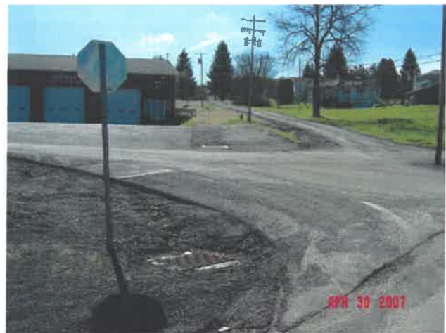
New Storm Drains and Catch Basins
