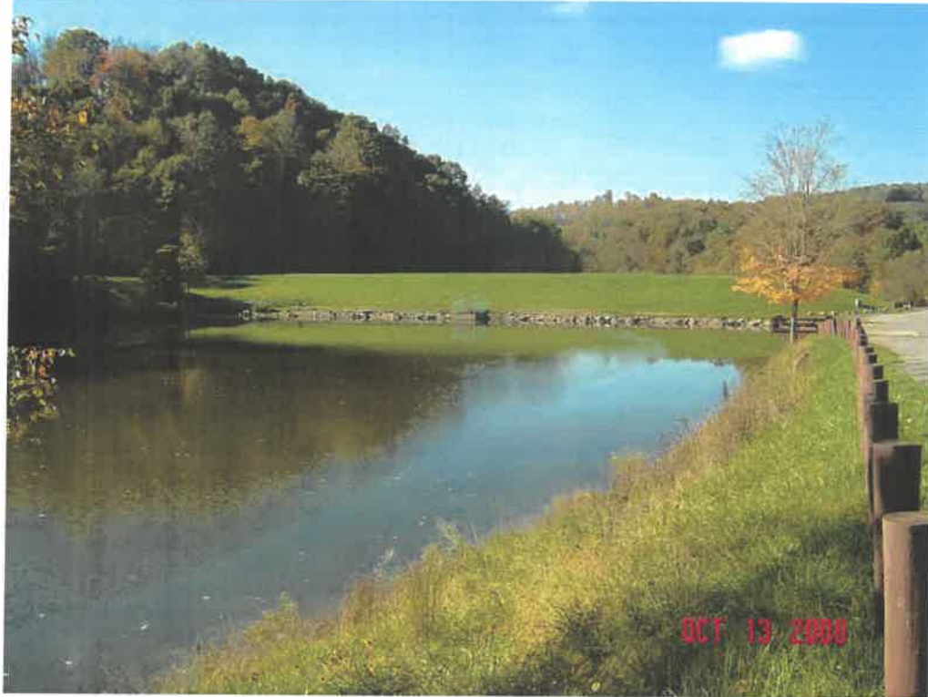
JIMMY LEWIS DAM MODIFICATION, MERCER CO., WV
