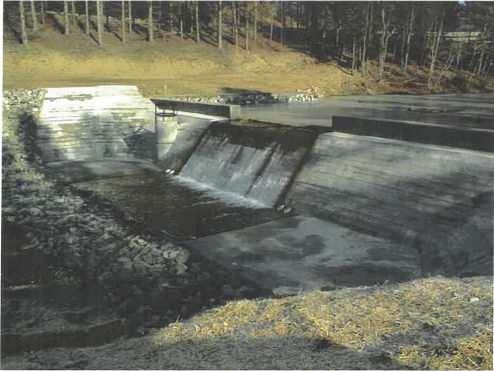
THOMAS DAM MODIFICATION, THOMAS, WV
