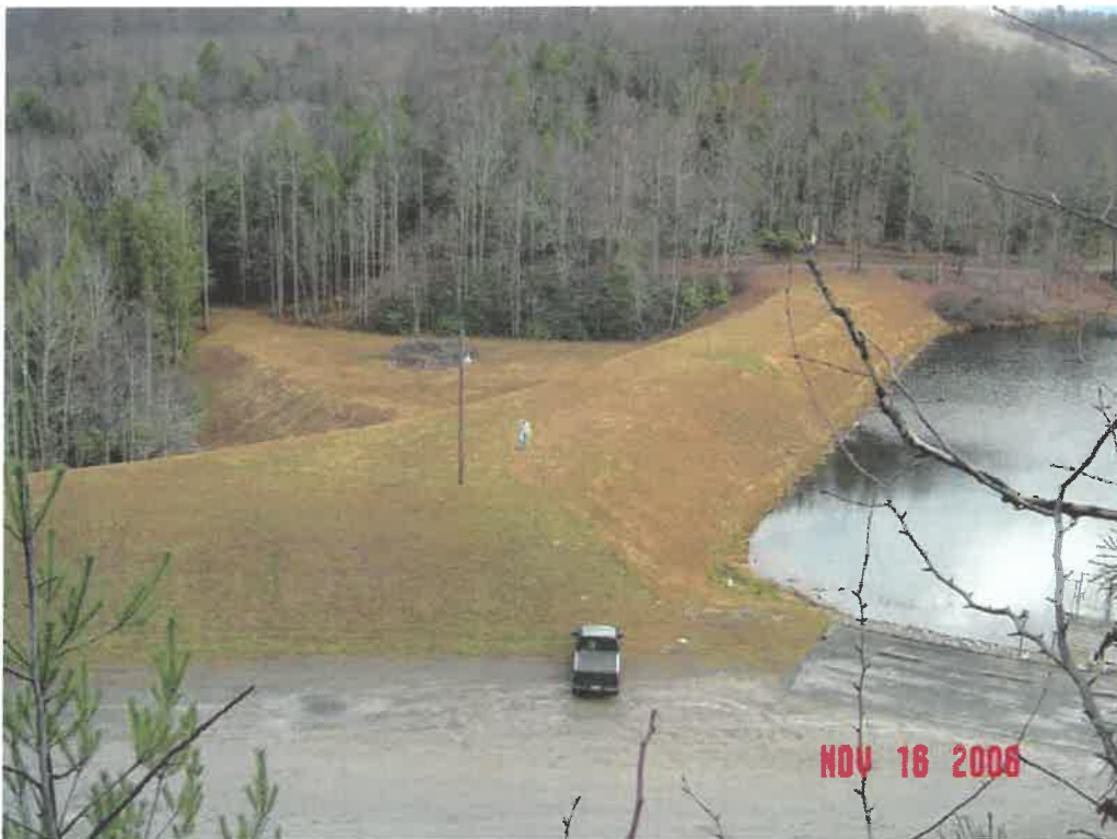
PLUM ORCHARD DAM MODIFICATION, FAYETTE CO., WV
