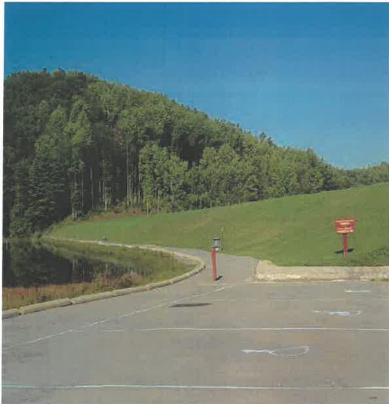
TETER CREEK DAM MODIFICATION, BARBOUR CO., WV
