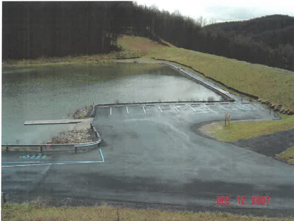
BAILEY DAM MODIFICATION, MONONGALIA CO., WV
