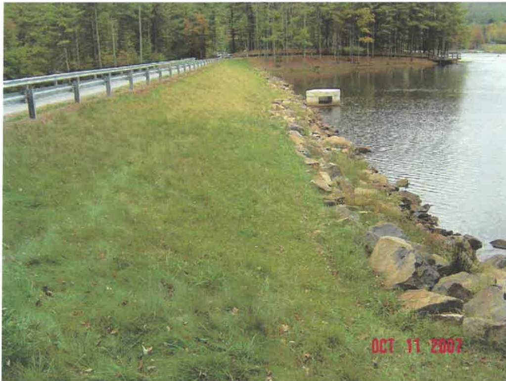
MONCOVE DAM MODIFICATION, MONROE CO., WV
