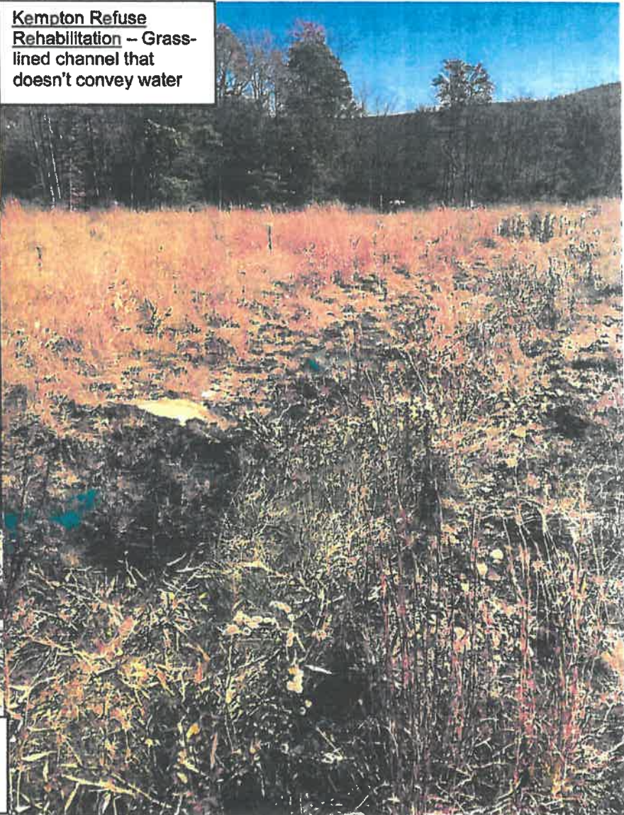
Kempton Refuse Rehabilitation – Erosion along grouted channel
