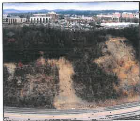
WVU Rockfall Project
