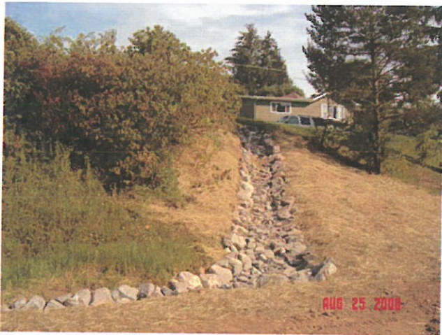
Erosion Repair – Rip Rap Armored Ditch
