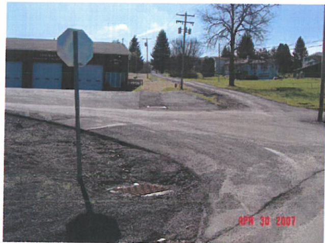
New Storm Drains and Catch Basins
