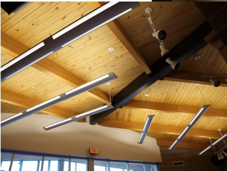
The main lobby framing consists of a tube steel beam, glulam beams and timber decking.
