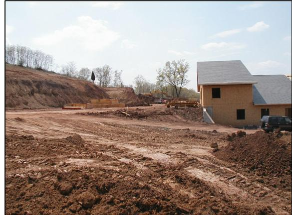
POTESTA prepared the topographic mapping for the project from ground survey information. The project included the design of four valley fills and a single side hill fill to accommodate approximately 740,000-cubic yards of excavated soil and rock.
