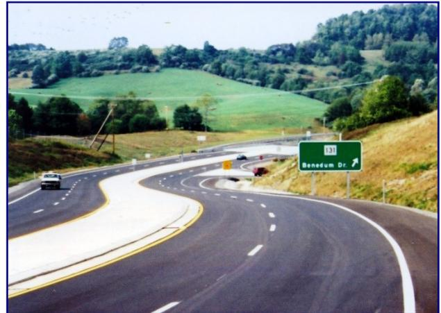
**Mineral Wells Industrial Park** – Construction and right-of-way plans were prepared for 0.65 mile of West Virginia Route 14/25 for access into the industrial park. Project also included determination of wetland impacts and development of a mitigation plan to account for wetlands lost as a result of construction.
