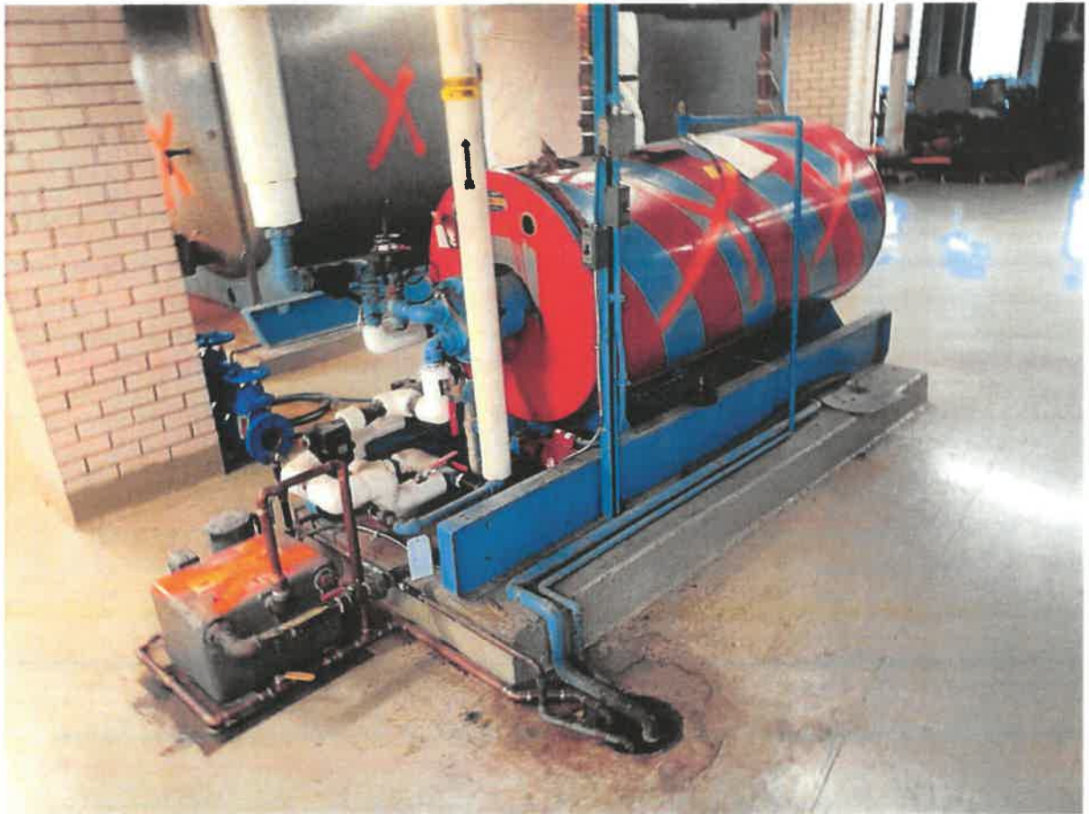
Exhibit D – Building 5 11th floor, pump station assembly for removal
