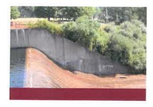
Our watershed hydrology and dam/spillway hydraulics analysis determined that the existing dam would only pass 58% of a PMP/6 hour design storm; therefore modifications to the existing dam/spillway would have to be made to safely pass the 70% PMP/6 hour design storm. In order to achieve that goal, Thrasher determined that the most efficient and economical solution would be to raise the dam to elevation and spillway to elevation 1031.0.
