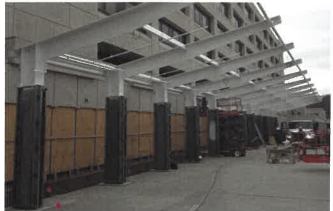
Recently completed is the New Front Entrance Canopy. Light and airy, this new design allows more daylight to enter into the building while expanding the drive lanes to 3.
