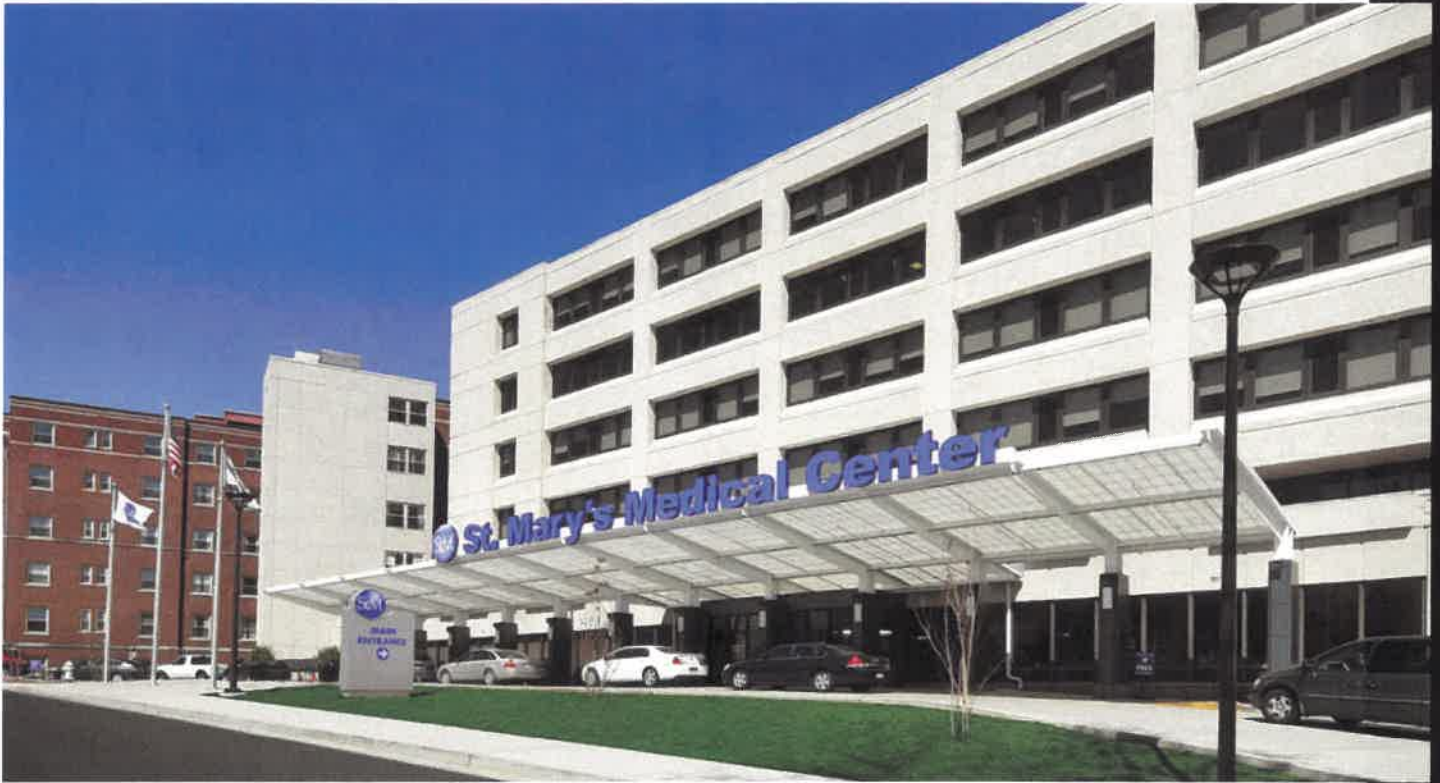
Recently completed is the New Front Entrance Canopy. Light and airy, this new design allows more daylight to enter into the building while expanding the drive lanes to 3.
