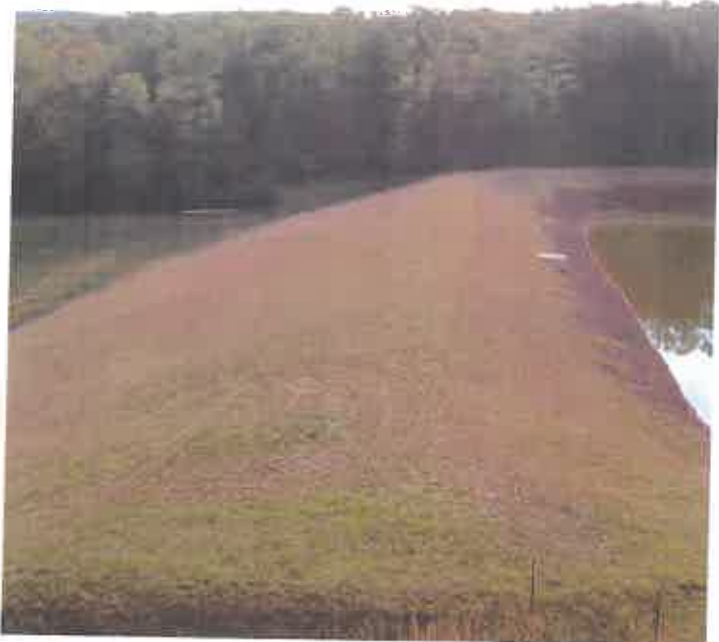
WILSON DAM MODIFICATION, HAMPSHIRE CO., WV
