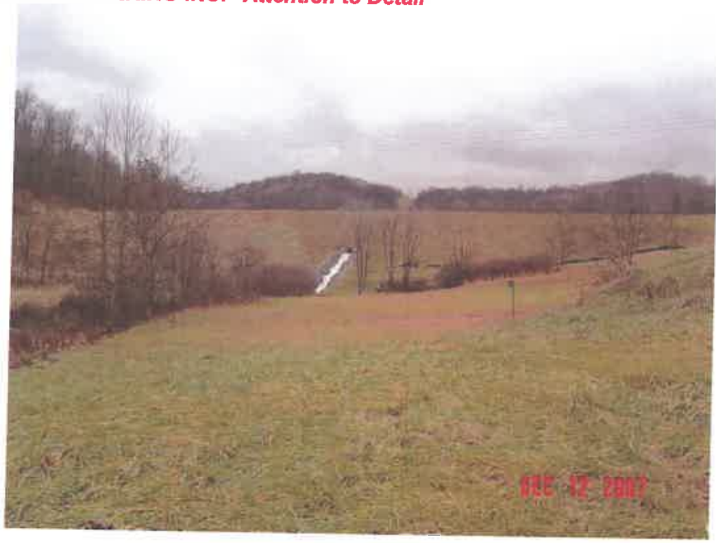
LEMLEY DAM MODIFICATION, MONONGALIA CO., WV
