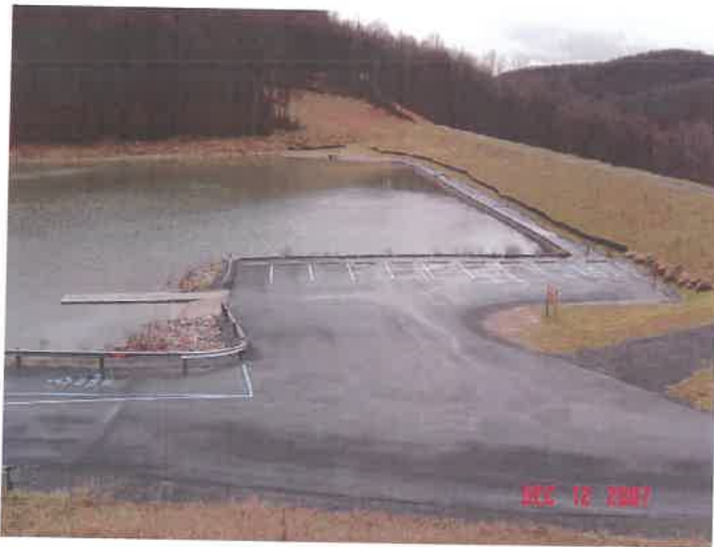
BAILEY DAM MODIFICATION, MONONGALIA CO., WV
