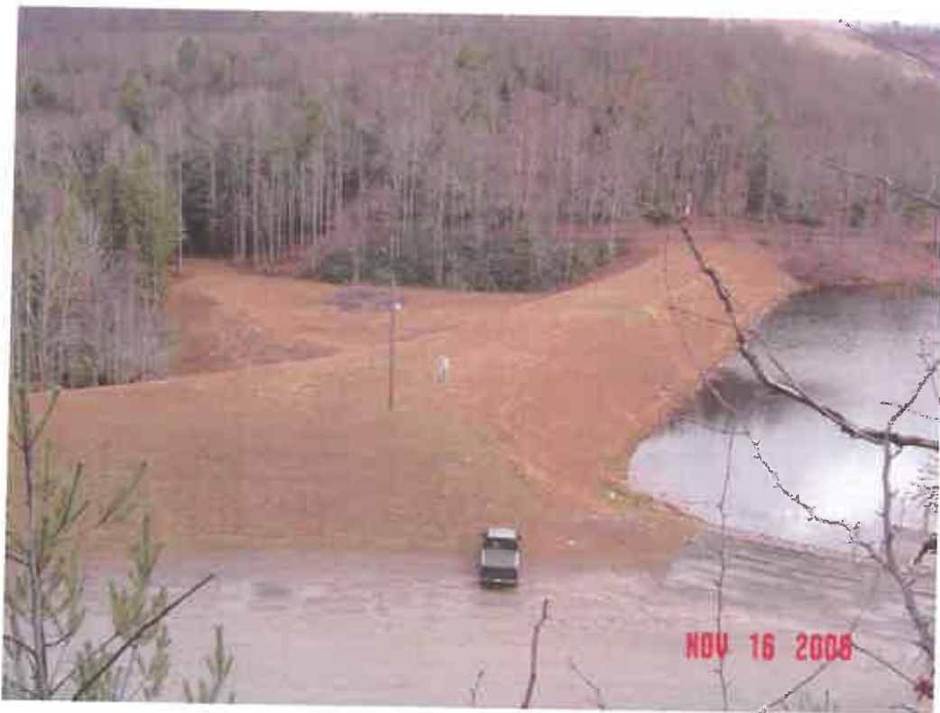
PLUM ORCHARD DAM MODIFICATION, FAYETTE CO., WV
