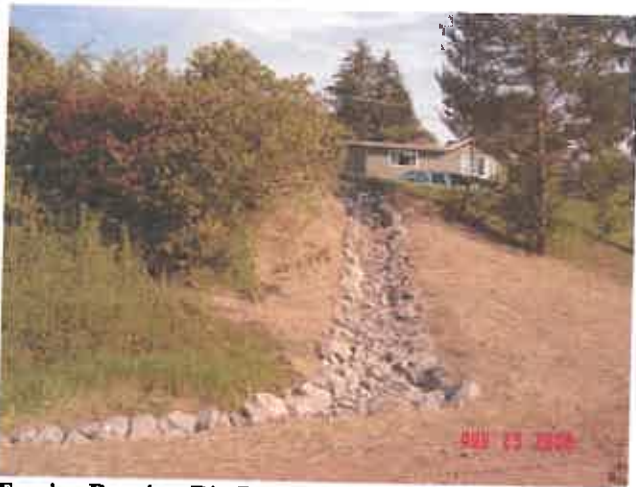
Erosion Repair – Rip Rap Armored Ditch
