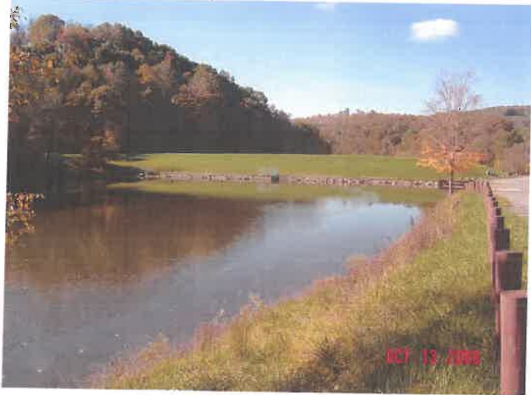
JIMMY LEWIS DAM MODIFICATION, MERCER CO., WV
