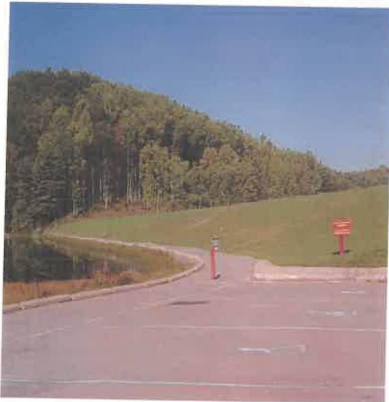
TETER CREEK DAM MODIFICATION, BARBOUR CO., WV
