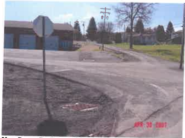
New Storm Drains and Catch Basins
