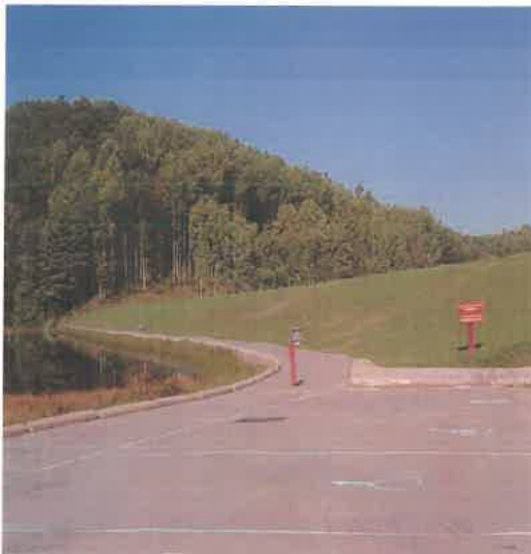
TETER CREEK DAM MODIFICATION, BARBOUR CO., WV
