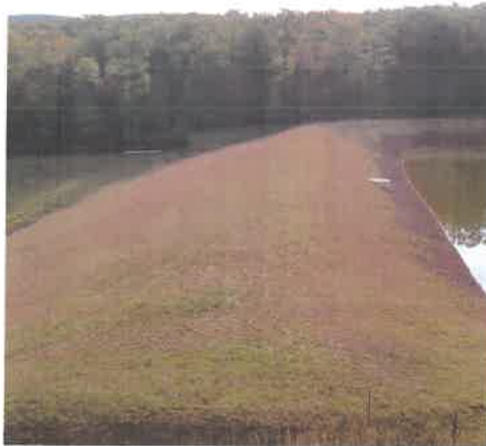
WILSON DAM MODIFICATION, HAMPSHIRE CO., WV
