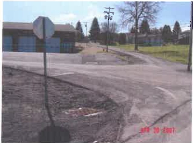
New Storm Drains and Catch Basins
