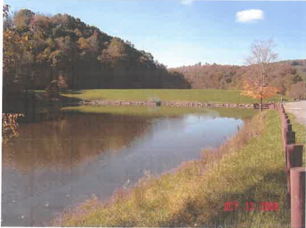
JIMMY LEWIS DAM MODIFICATION, MERCER CO., WV
