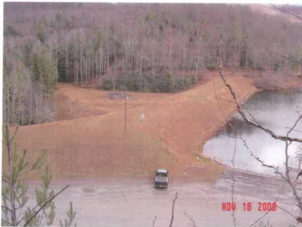
PLUM ORCHARD DAM MODIFICATION, FAYETTE CO., WV
