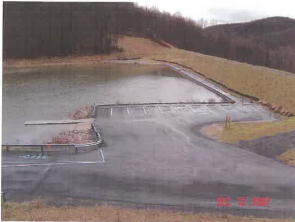
BAILEY DAM MODIFICATION, MONONGALIA CO., WV
