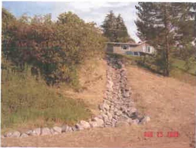
Erosion Repair -- Rip Rap Armored Ditch
