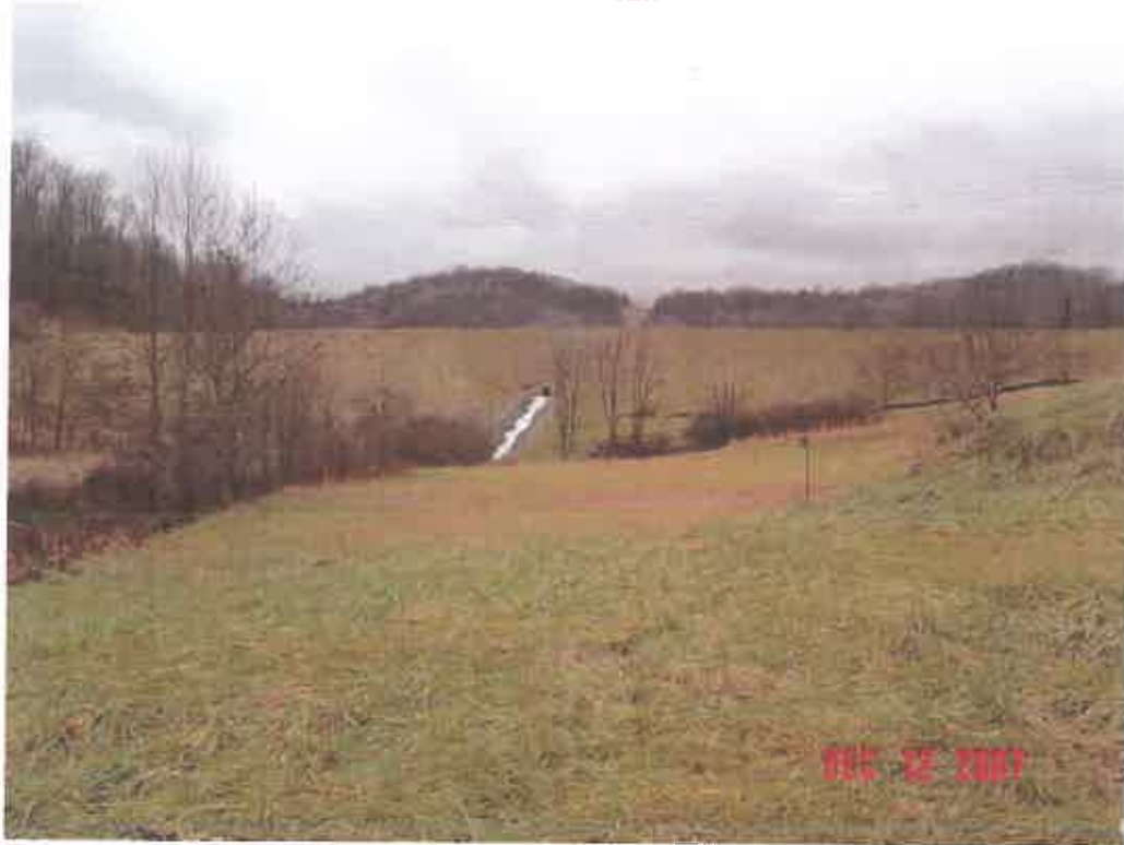
LEMLEY DAM MODIFICATION, MONONGALIA CO., WV
