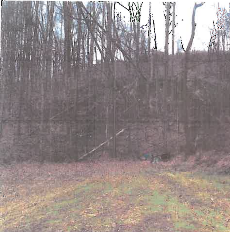
Camden (Wilson) Landslide – Slide mass from behind Wilson residence, showing downed trees
