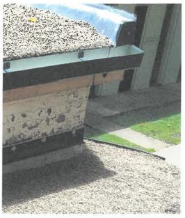
West Virginia Division of Natural Resources contracted Montum Architecture to specify and administer roofing replacement of the Pool Bathhouse at Berkeley Springs State Park. The existing roofing was a combination of EPDM and built-up roofing. Failing wood framing was replaced and ACM abatement was incorporated in the demolition.
