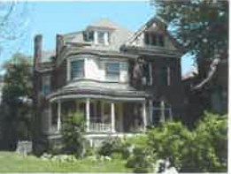
304 South Front Street Wheeling, WV (in Wheeling Island Historic District - NRHP#: 92000320) Customer: McKinley Architecture and Engineering Project Cost: $275,000
