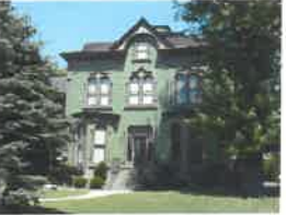
400 South Front Street Wheeling, WV (in Wheeling Island Historic District - NRHP#: 92000320) Customer: McKinley Architecture and Engineering Project Cost: $250,000
