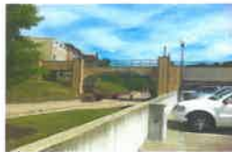
Fairmont State University Parking Garage Pedestrian Bridge Fairmont, WV
