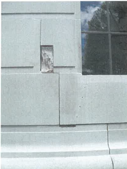
Other repairs included various spall repairs, pinning and epoxy injection of larger cracks and lifting and pinning keystones over windows.
