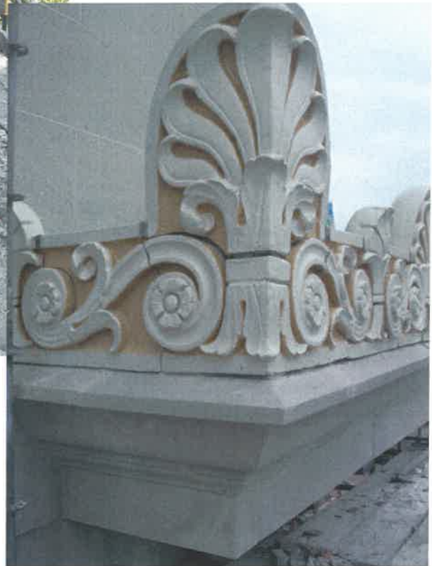
Portions of the limestone cornice were damaged to the point that they fell when work was being conducted and had to be pinned back in place.
