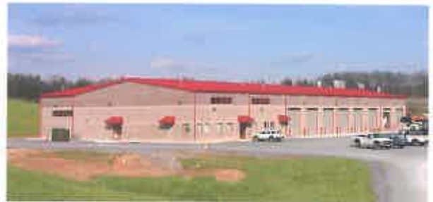
District Seven Office Building & Equipment Shop will be underconstruction by end of 2018
