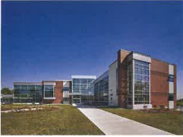
Middlesex County College New South Hall Science Building Edison, NJ
