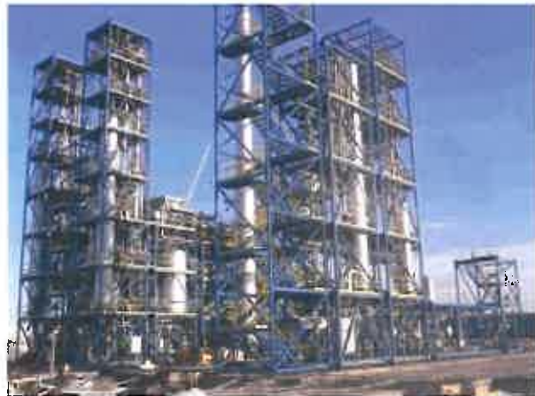
Polysilicon Production Facility Qujing, China
