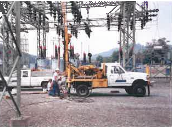
GenOn Northeast Management Company Five-phased development of an ash disposal site Shawville, PA
