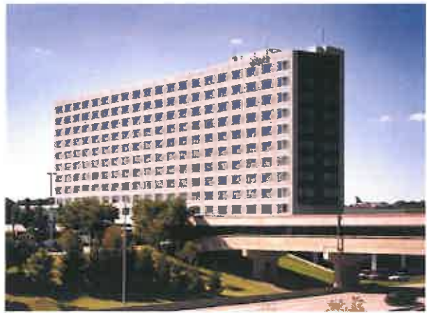
Hyatt Hotel at the Pittsburgh International Airport Dauphin County General Authority Pittsburgh, PA
