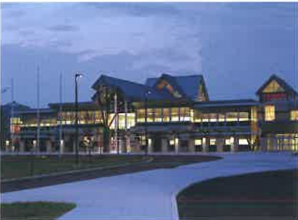
New Central York High School York, PA
