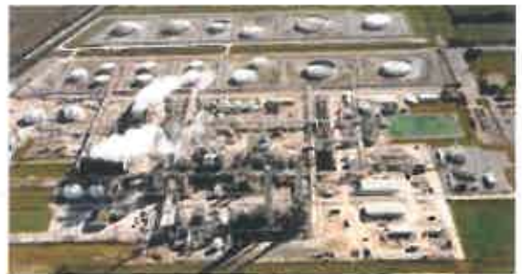
COSMAR Modernization Project Carville, LA
