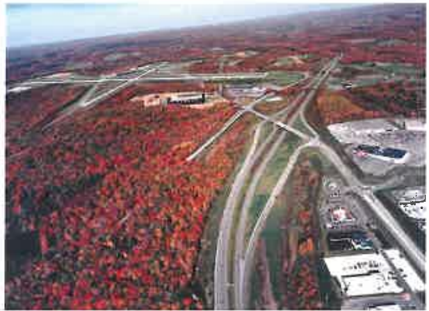
Johnstown Galleria Interchange Johnstown, PA
