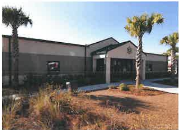
Chatham County, GA Detention Center Campus Upgrades Savannah, GA
