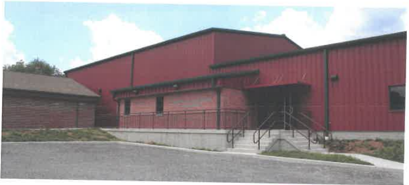
New Pocahontas County Wellness Center Marlinton, West Virginia
