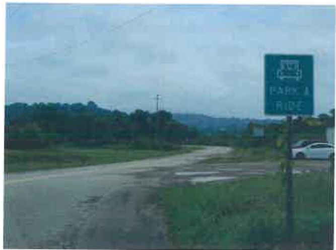
Looking East on CR 68/2 through Site Location
