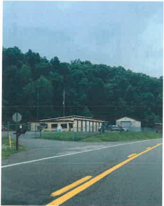
Existing Medina Substation
