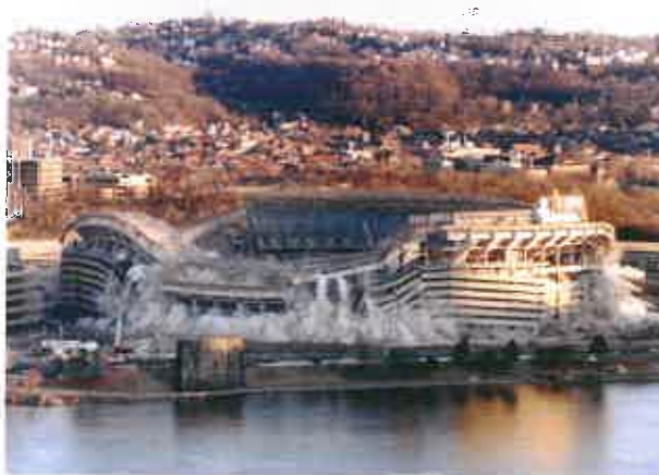
Demolition of Three Rivers Stadium & Engineering Services for Heinz Field Pittsburgh, PA
