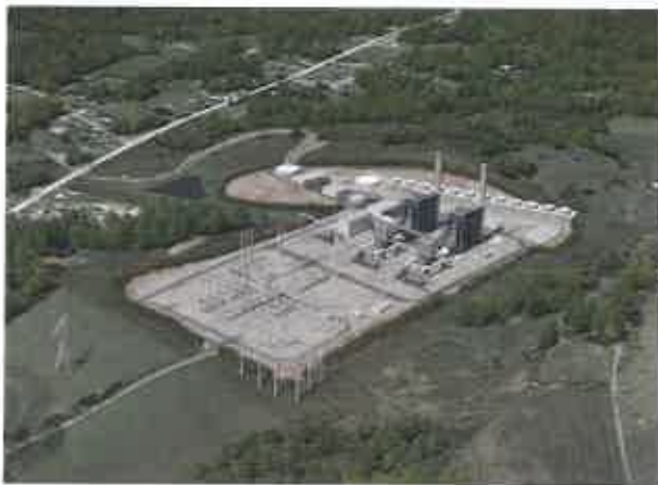
Competitive Power Ventures (CPV) CPV Fairview Energy Center Vinco, Jackson Township, Cambria County, PA
