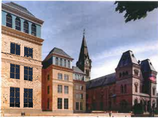
Blair County, PA Courthouse Renovations/Additions Hollidaysburg, PA
