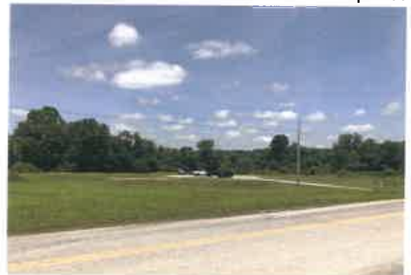
West Virginia Division of Highways District 3, New I-77 Medina Substation
