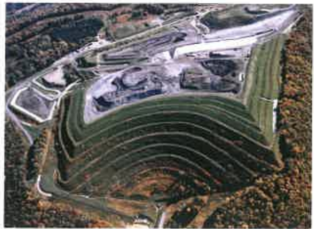
Shawville Power Plant Ash Disposal Site Clearfield, PA
