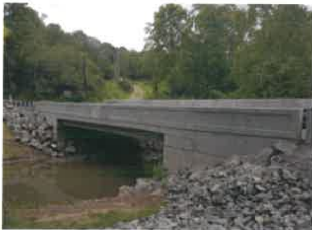
Rapid Bridge Replacement P3 Project 12 Bridge replacements across Districts 11-0, 12-0, 10-0, 2-0, 9-0, 8-0, and 6-0
