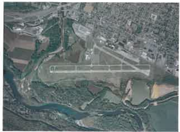
Williamsport Municipal Airport Authority Runway 9-27 Approach Improvements & Rehabilitation Williamsport Regional Airport, Montoursville, PA
