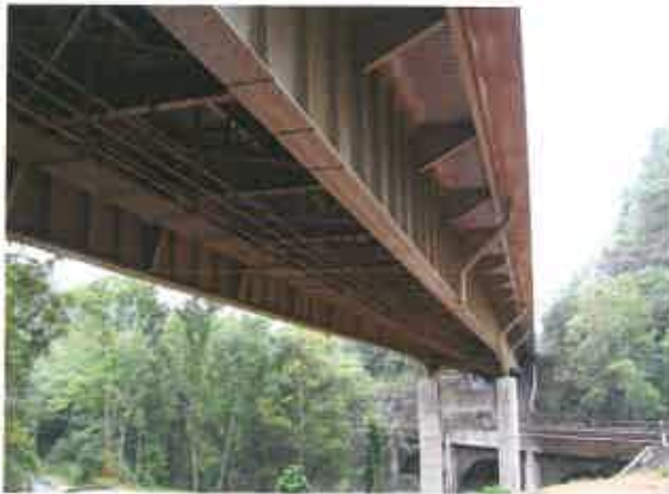
PennDOT, District 9-0 Pemberton Bridge Rehab Warriors Mark Township, PA
