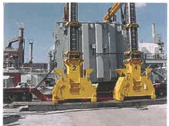
Power System Expansion Convent, LA
