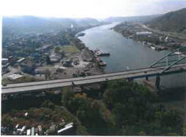
West Virginia Department of Highways I-470 Approach Bridge Rehabilitation City of Wheeling, Ohio County, WV
