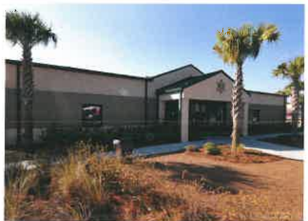
Chatham County, GA Detention Center Campus Upgrades Savannah, GA
