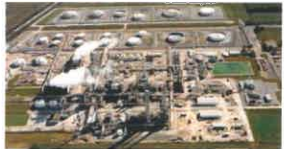
COSMAR Modernization Project Carville, LA
