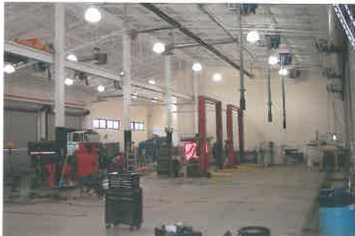
Equipment Maintenance Shop
