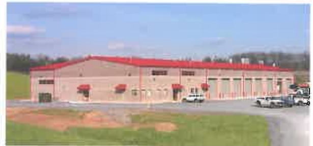
District Seven Office Building & Equipment Shop will be underconstruction by end of 2018
