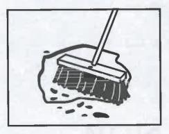
PREPARE: Remove all loose dust, dirt and debris by sweeping with a broom.
