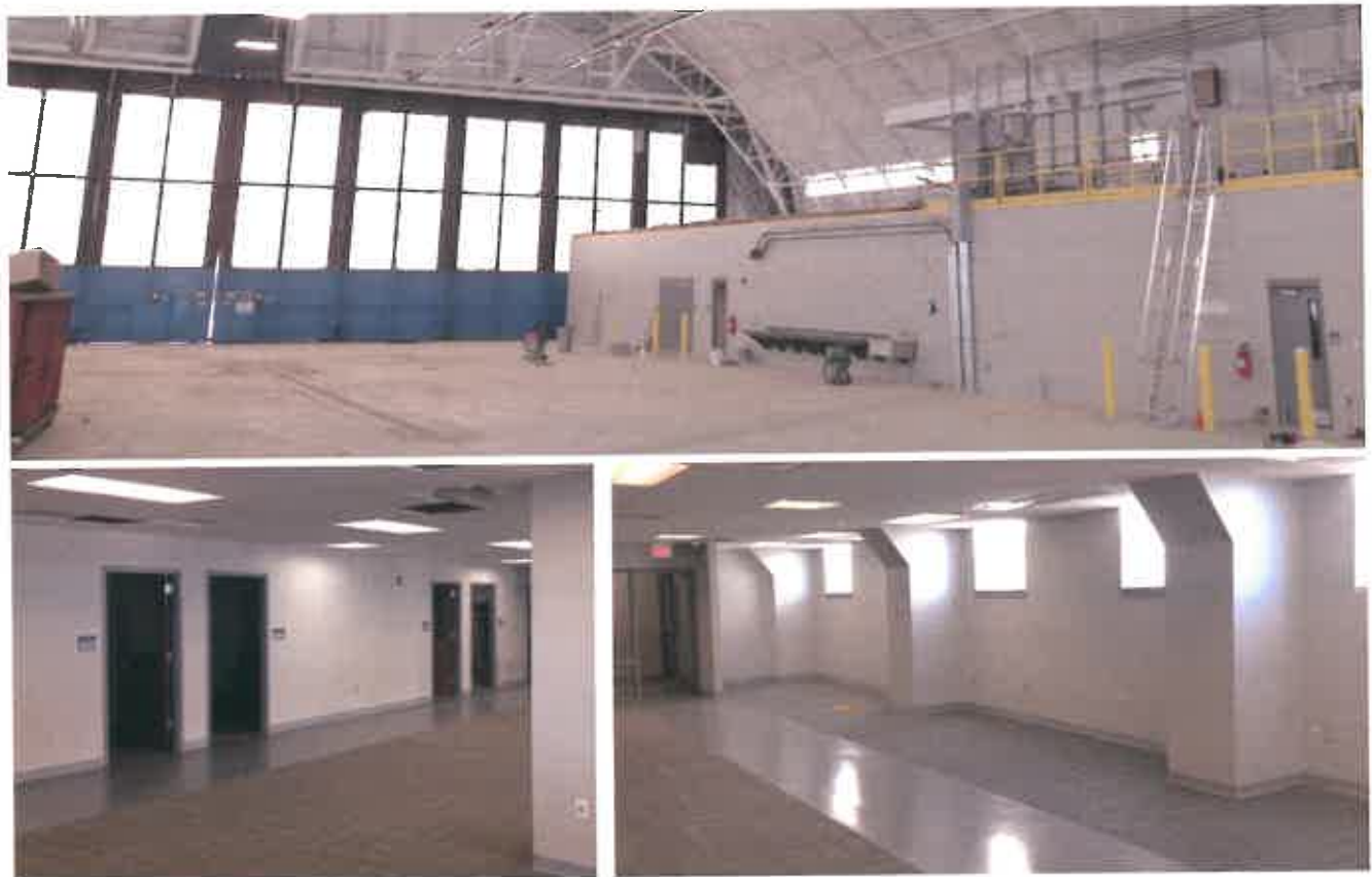
GRW provided design and construction phase services for the WV ANG's 130 th Airlift Wing Building 107 Renovation. With a construction budget of $5M, the awarded bid was $4,941,290, and the final construction cost was $4,991,876 (within 1% of awarded bid).
